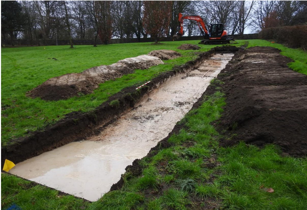
Plate 3: Showing evaluation Trench 1. Looking south with two-metre scale inside the trench.
