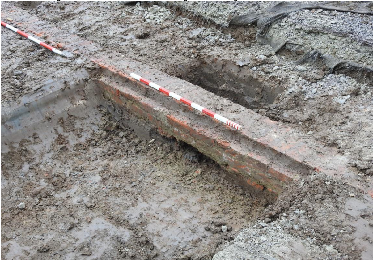
Plate 16: Showing exposed retention wall in Trench 8A. Looking south-east with one-metre scale.
