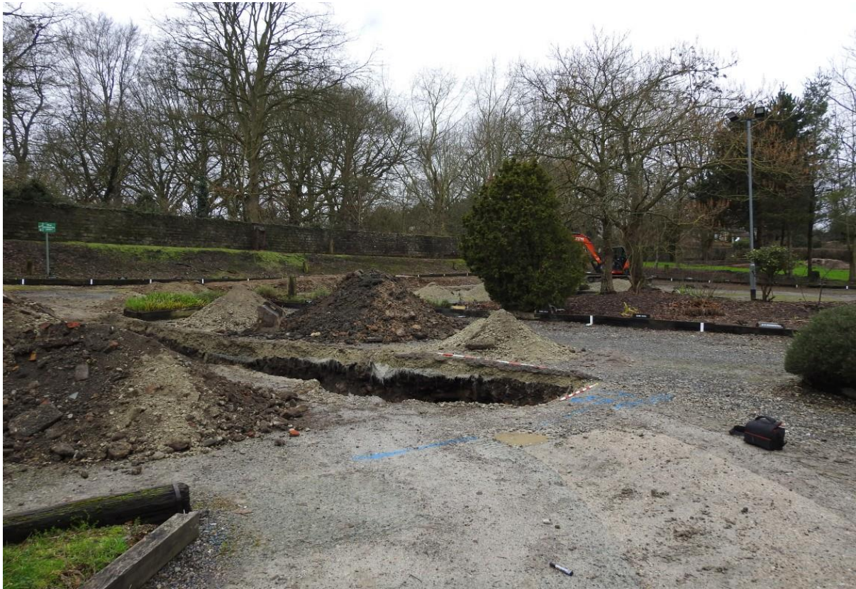
Plate 1: The site looking south-west.
